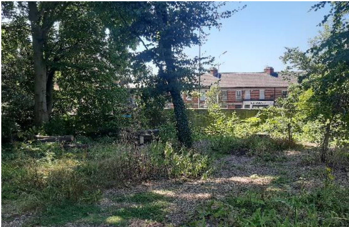
Rathfarnham Castle Park where retaining walls are present.
